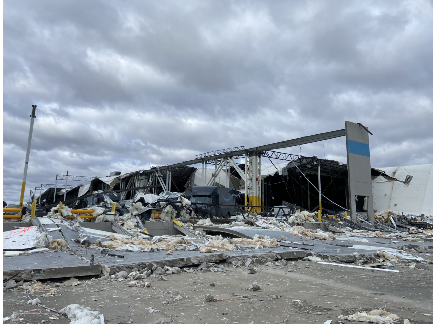
Damage at an Amazon facility in Edwardsville, Illinois. Photo by NWS St. Louis.
