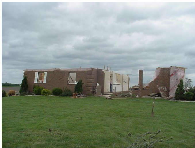
Tornado Damage to brick home in Ely, Missouri
