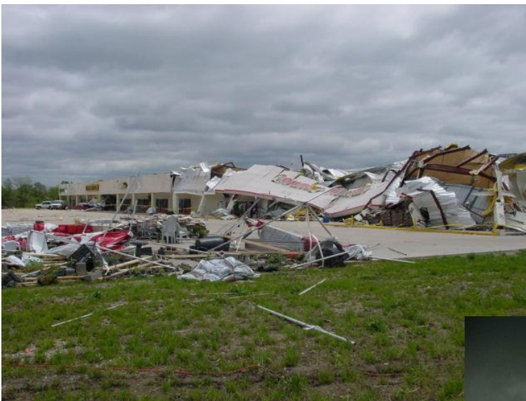
Tornado Damage to County Market in Canton, MO
