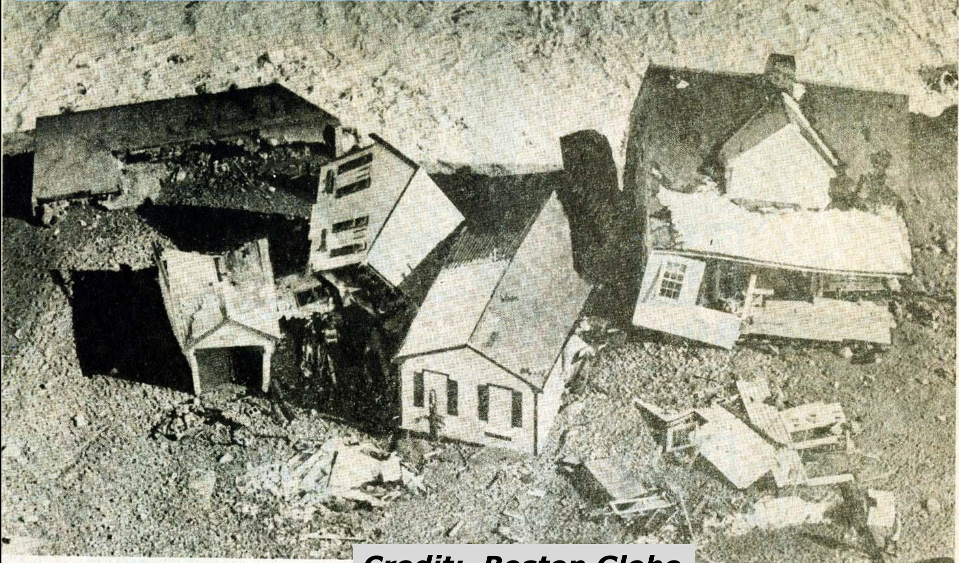
Sea-ravaged houses along Peggoty Beach in Scituate.
